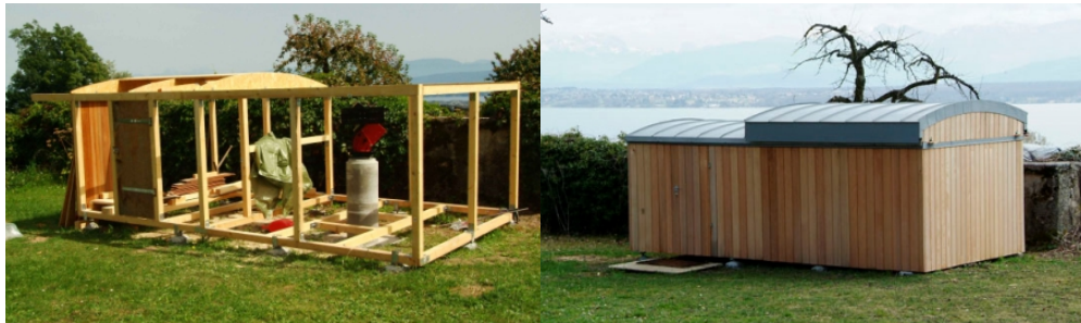
Left: frame and column with 1 m3 concret in the ground. Right: finished observatory with sliding roof.
